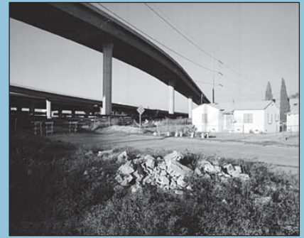
The Century Freeway Project cut directly through whole neighborhoods, forcing over 21,000 people to relocate. CEQA ensured that these people had substantial relocation assistance.
