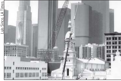
Historic St. Vibiana's Cathedral (above), in downtown LA, was saved from demolition by CEQA. It will be adaptively reused as a performing arts venue. Read more on page 157.
