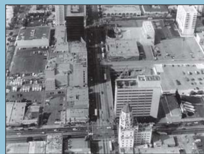
Hollywood & Highland Site Before Construction
